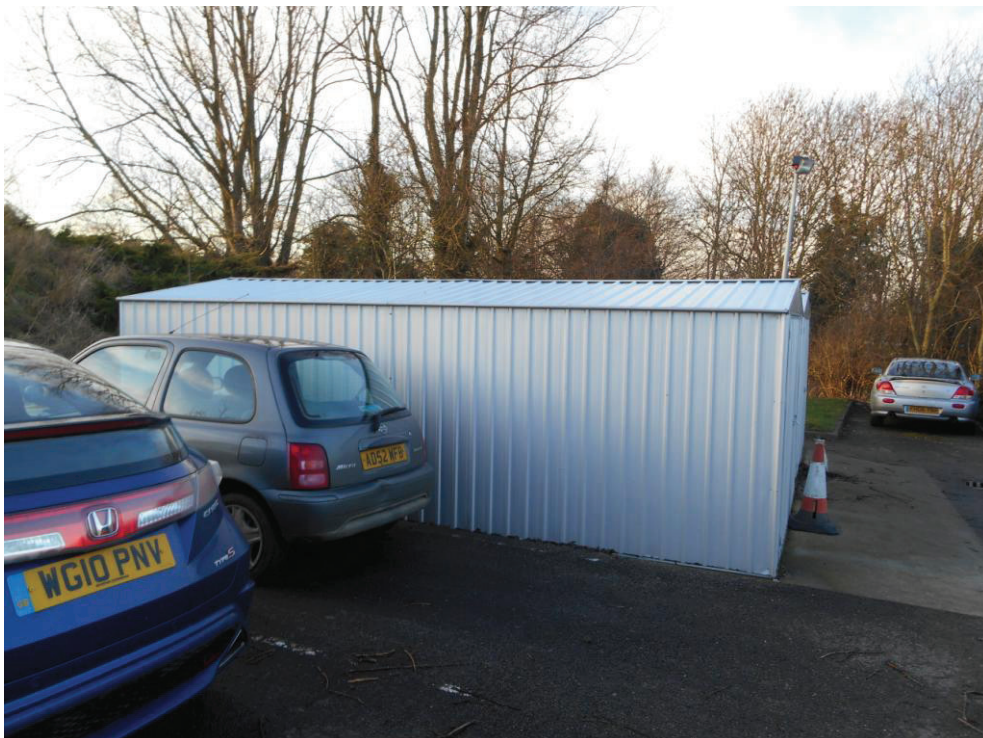
South Side of Garages
