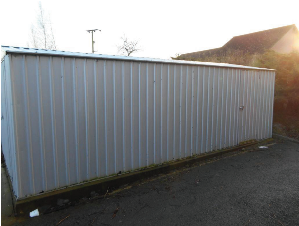
North side of Garages
