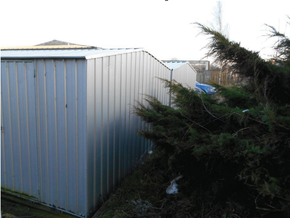
Rear of Garages
